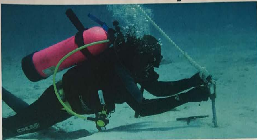
Diver secures mooring down-line.
